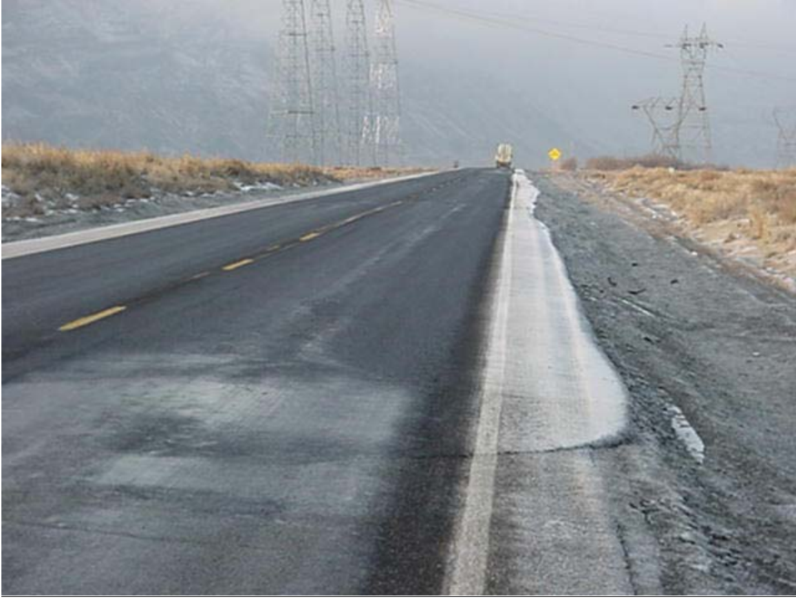
Photo 3. Close up of ice on shoulder just outside of application area.
