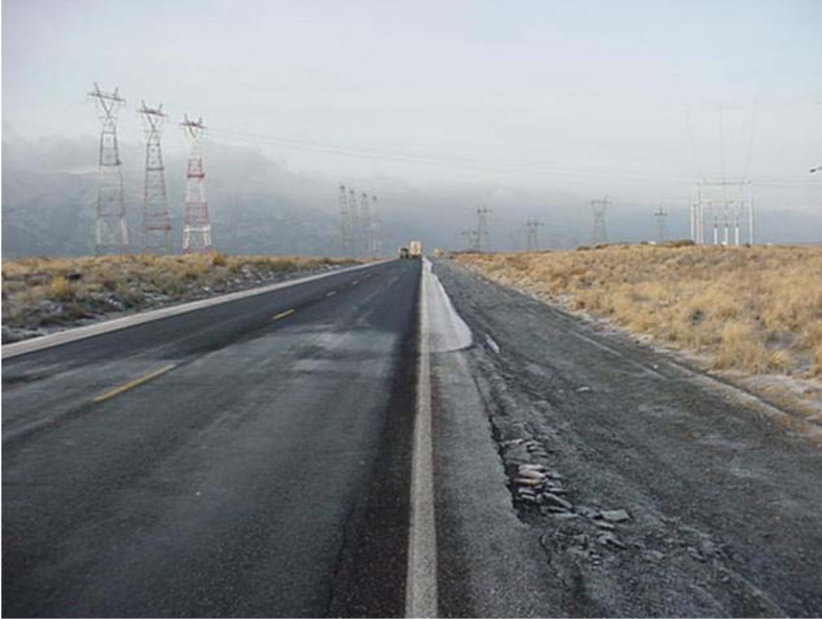
Photo 2. Note ice on shoulders and edge of roadway near edge lines. Just outside of the application area.
