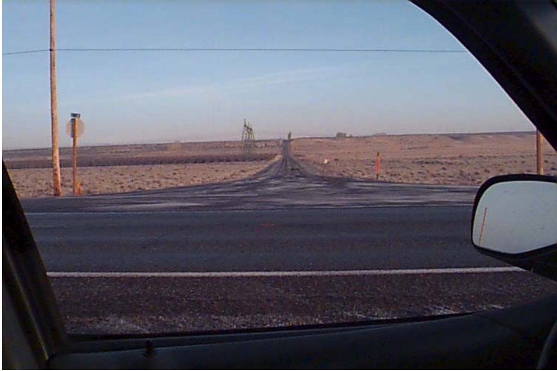
Photo 7. Untreated and icy side road.
