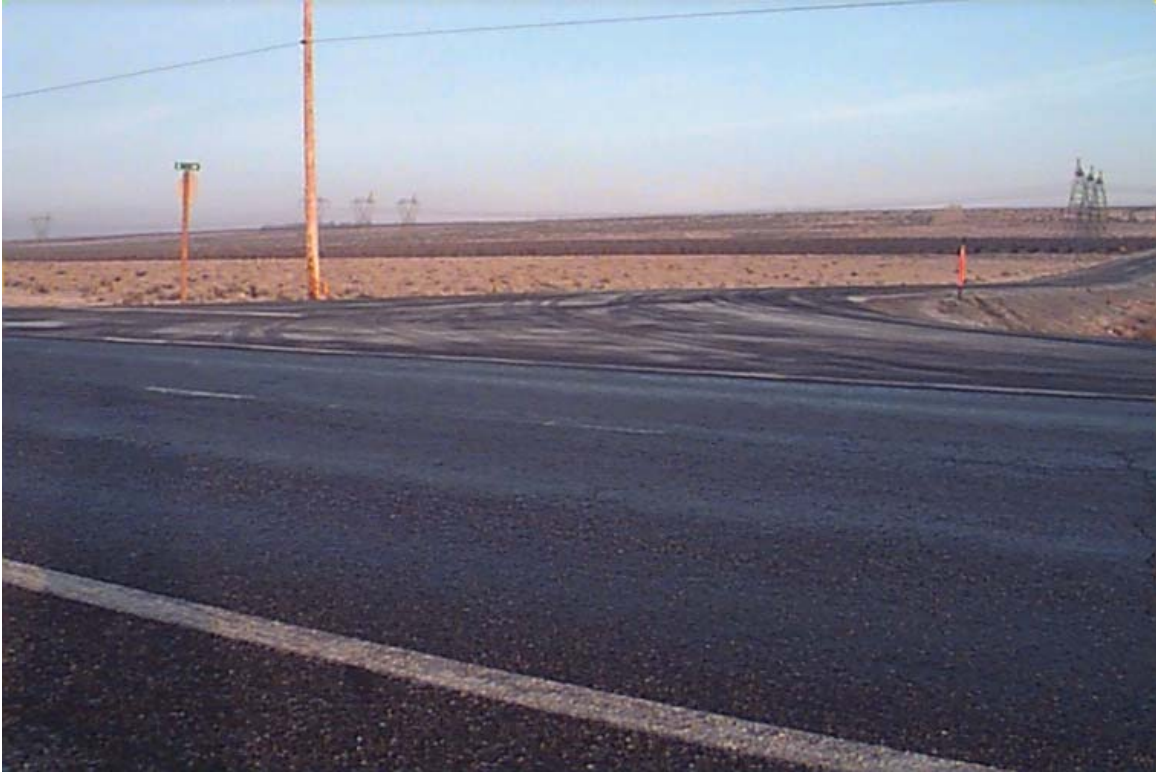
Photo 6. Note ice on untreated side road. Also note tracking of material and melting action on the side road.
