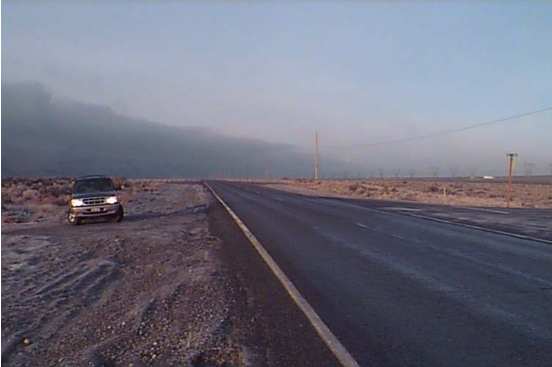
Photo 5. Note ice on side road that was untreated.
